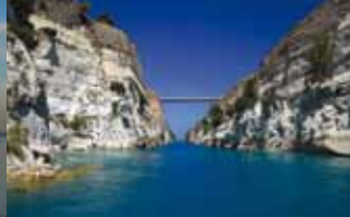
Corinth Canal, Greece
